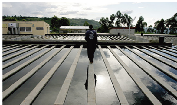
A WATER TREATMENT PLANT TO COMBAT CHOLERA KALEMIE, DRC
